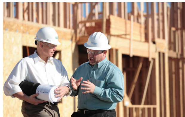
MEETING OF MINDS: Sales rep Mike Rasmussen (l) meets on the job site with Ray Ferrarini of Shea Homes, which is using iLevel material to build 300 new homes.
